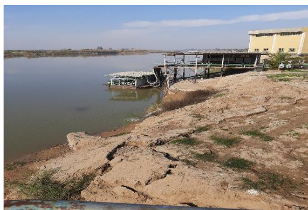
Fig.1: A view of the water catchment pond and its equipment
